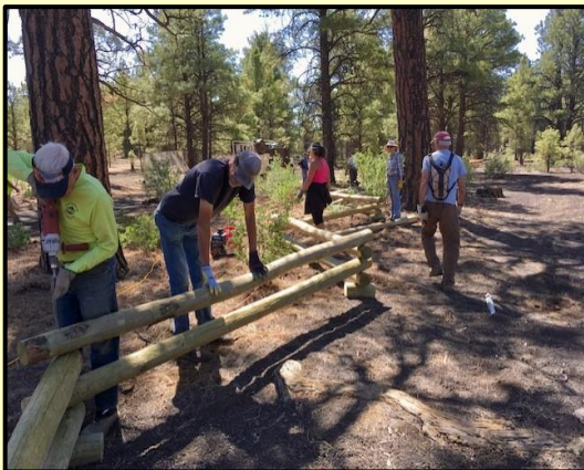
Log worm fence construction at Cinder Hills
