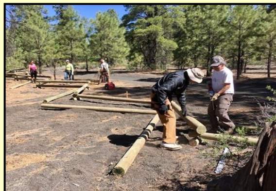
Log worm fence construction at Cinder Hills
