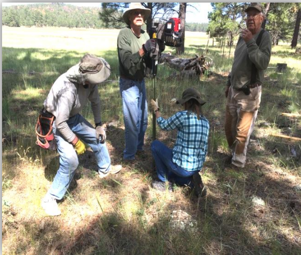
Placing T-post for new fence
